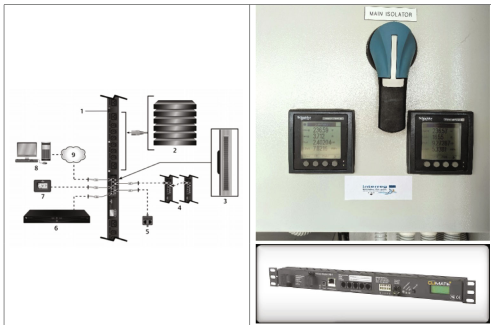
FIGURE 6 Indoor electricity and climate sensors.
